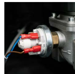
Gas inlet low pressure switch
