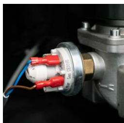
Gas inlet low pressure switch
